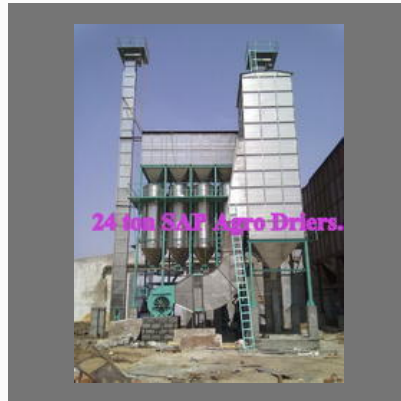
Paddy Parboiling Plant
